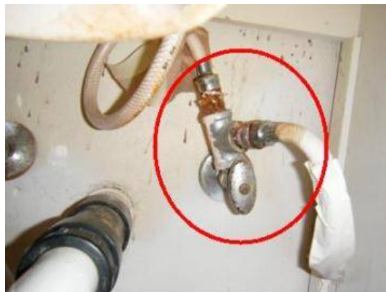
Water is leaking at the left sink's cold water angle stop valve.
