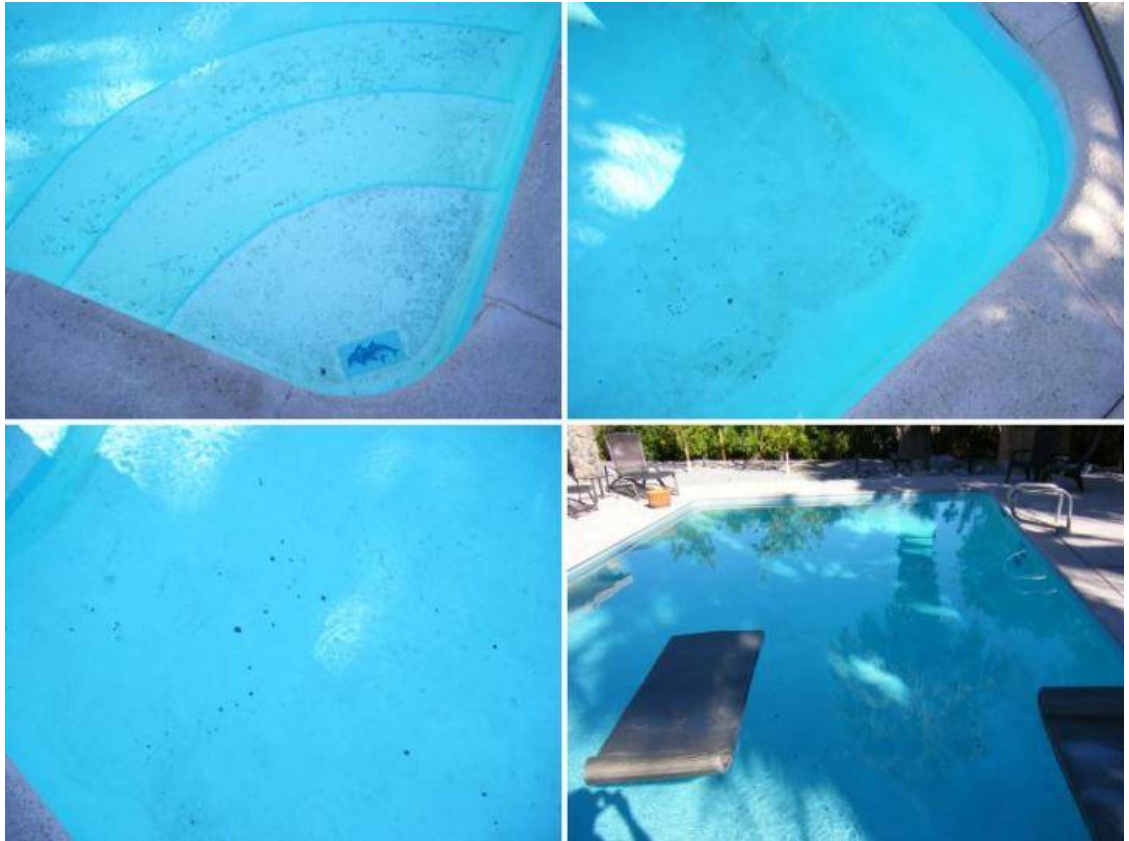
Surface is in poor condition, with several chipped areas of plaster noted.
