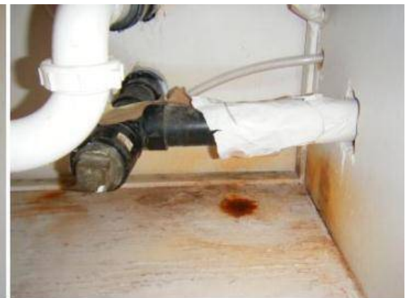
Water is leaking at the left sink's cold water angle stop valve.
