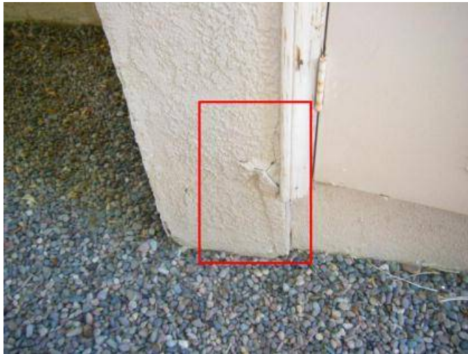
There are two holes cut into the stucco of the East mechanical closet and damaged stucco at the bottom-left of the mechanical room doors.
