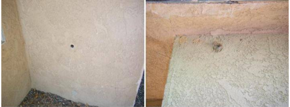
There are two holes cut into the stucco of the East mechanical closet and damaged stucco at the bottom-left of the mechanical room doors.
