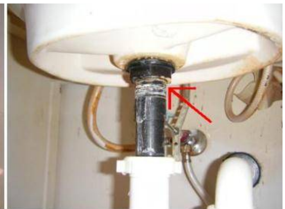
The left sink is cracked and leaks water at the sink's connection to the drain.
