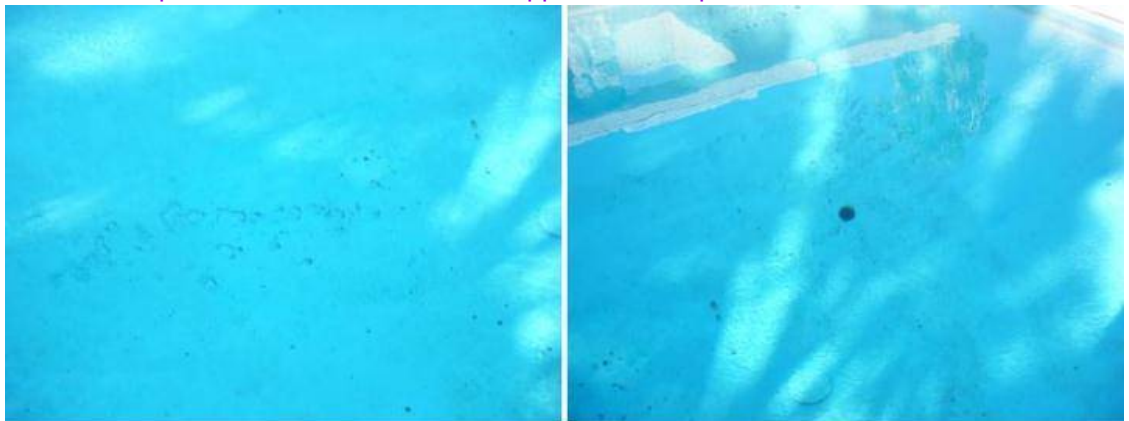
Surface is in poor condition, with several chipped areas of plaster noted.
