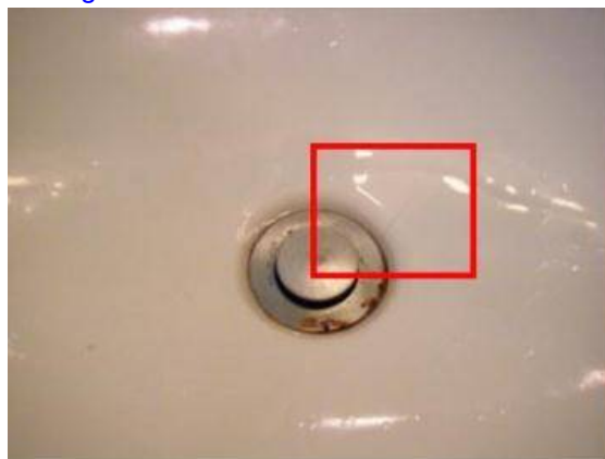
The left sink is cracked and leaks water at the sink's connection to the drain.
